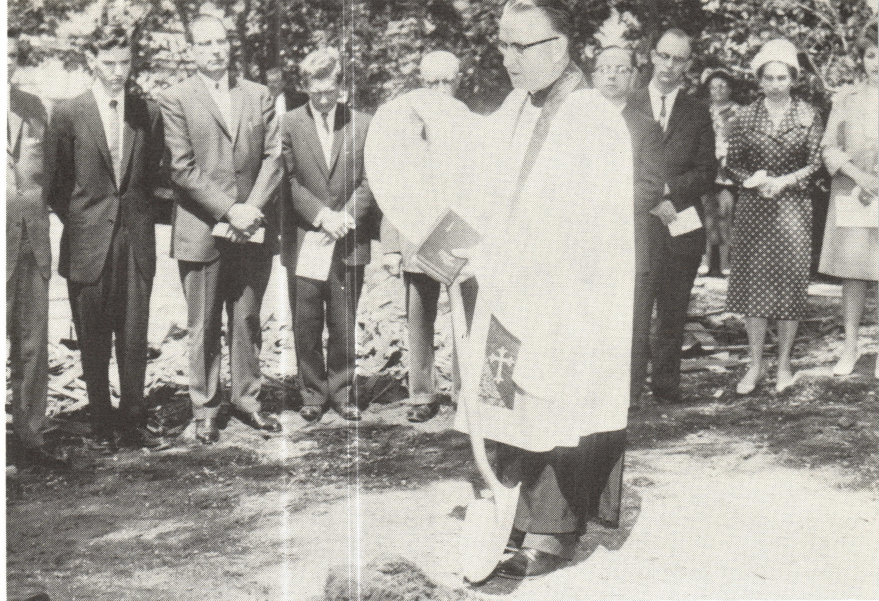
Ground Breaking of New Church
